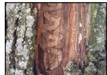
Insect damage (tunneling)
